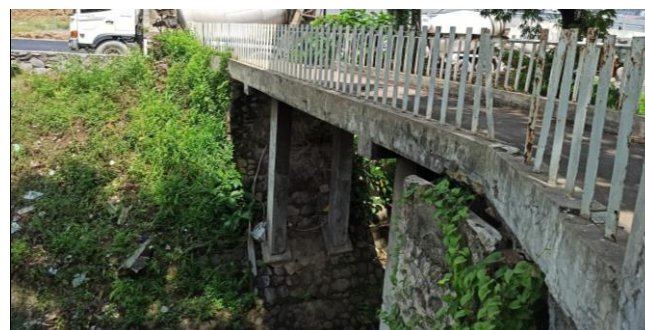
TAMPAK SAMPING KIRI
