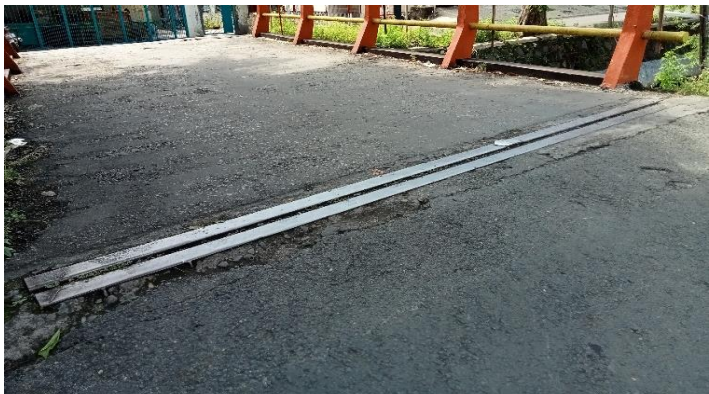
KONDISI EXPANSIONT JOINT
