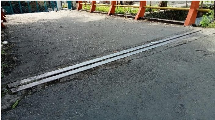
KONDISI EXPANSIONT JOINT
