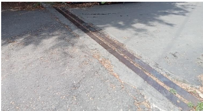
KONDISI EXPANSIONT JOINT
