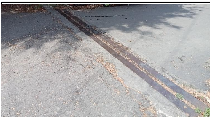
KONDISI EXPANSIONT JOINT
