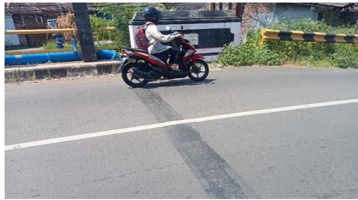
KONDISI EXPANSIONT JOINT
