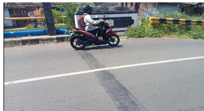
KONDISI EXPANSIONT JOINT
