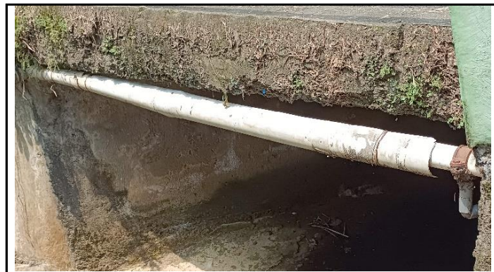
PIPA UTILITAS AIR MINUM
