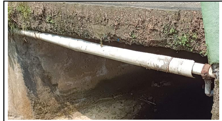
PIPA UTILITAS AIR MINUM
