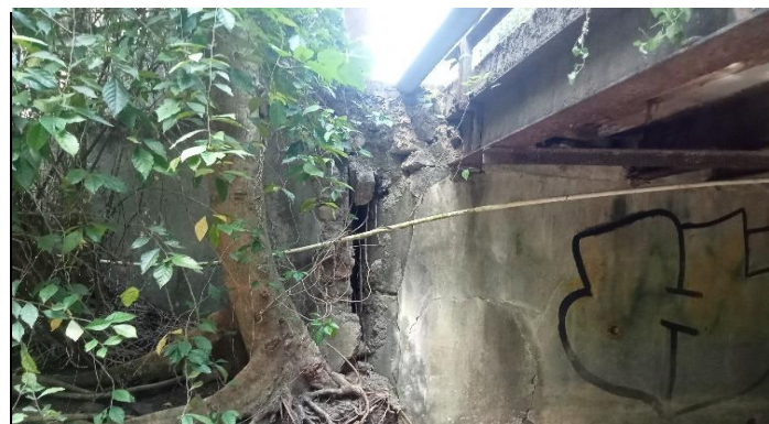
DIDNDING PENAHAN TANAH PECAH
