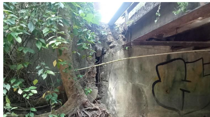
DIDNDING PENAHAN TANAH PECAH
