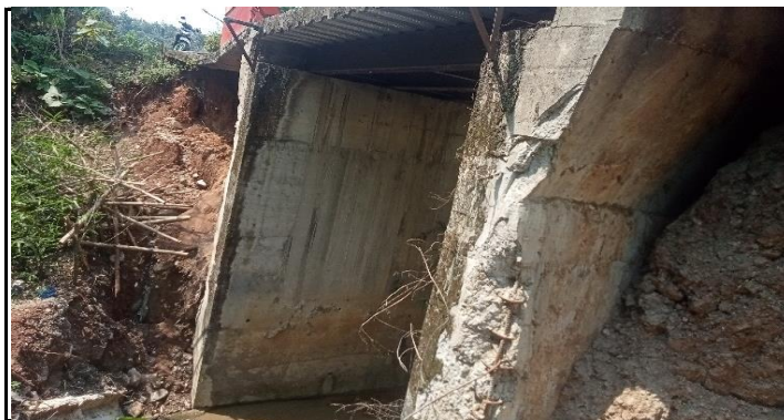
DINDING PENAHAN TANAH LONGSOR
