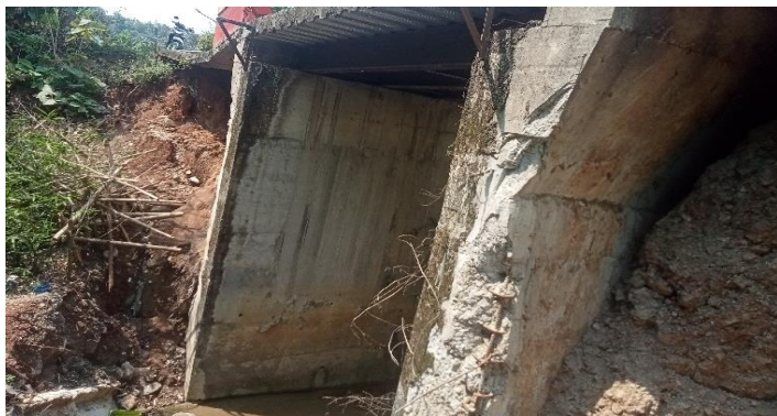
DINDING PENAHAN TANAH LONGSOR
