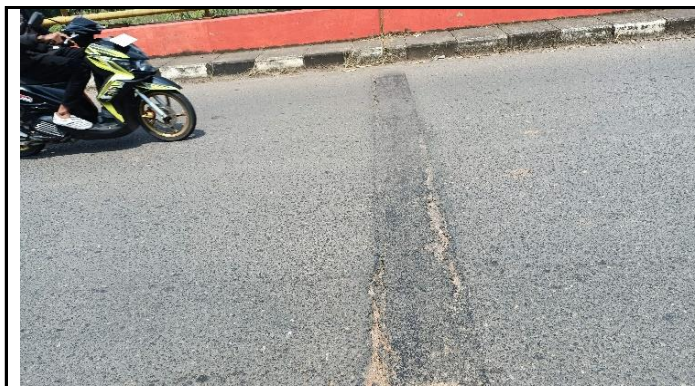
SAMBUNGAN SIAR MUAI (EXPANTION JOINT)
