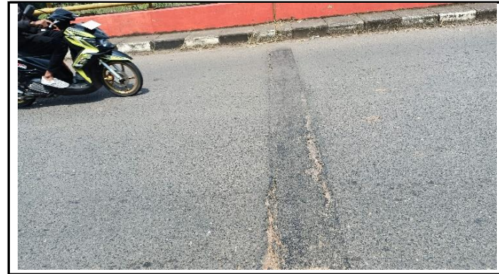
SAMBUNGAN SIAR MUAI (EXPANTION JOINT)
