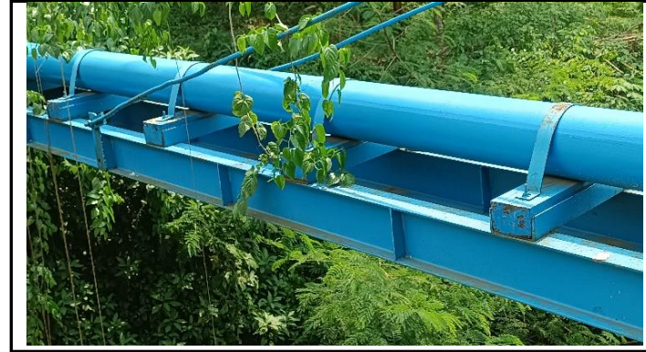
PIPA UTILITAS AIR MINUM
