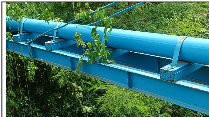
PIPA UTILITAS AIR MINUM
