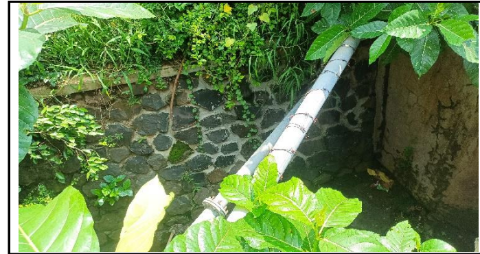
PIPA UTILITAS AIR MINUM
