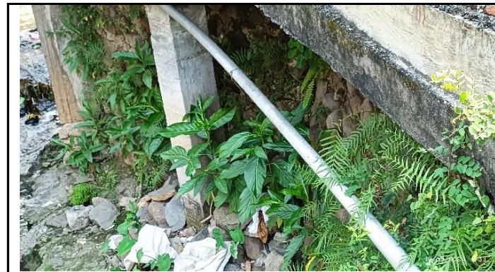
PIPA UTILITAS AIR MINUM
