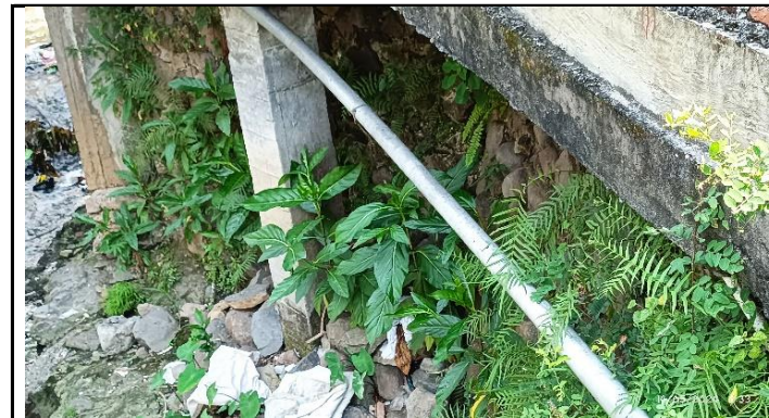
PIPA UTILITAS AIR MINUM
