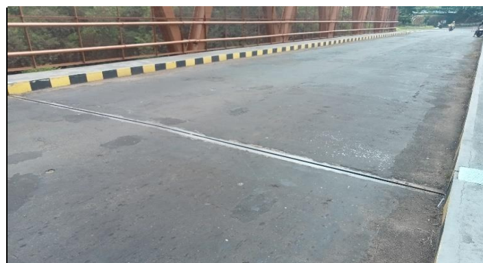
KONDISI EXPANSIONT JOINT
