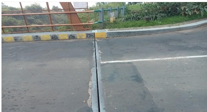
KONDISI EXPANSIONT JOINT
