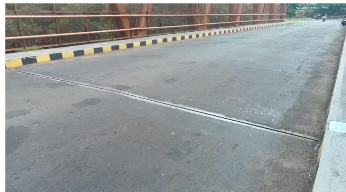
KONDISI EXPANSIONT JOINT
