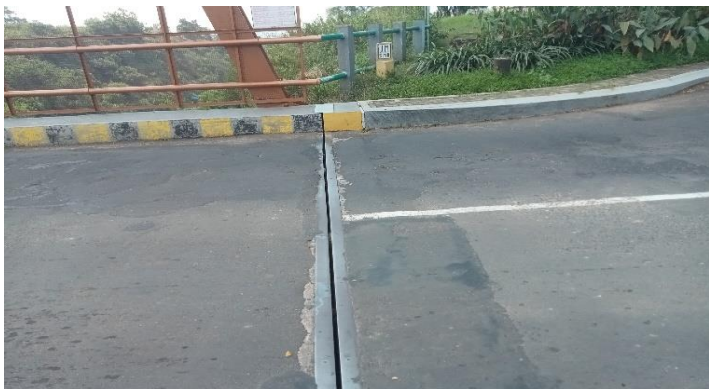
KONDISI EXPANSIONT JOINT
