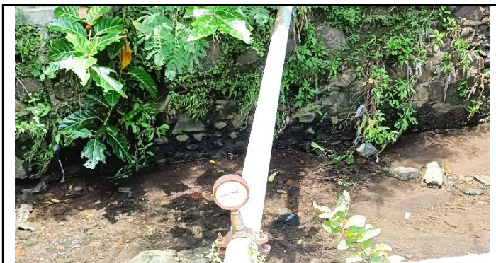
PIPA UTILITAS AIR MINUM
