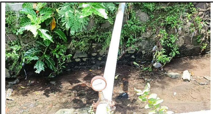
PIPA UTILITAS AIR MINUM
