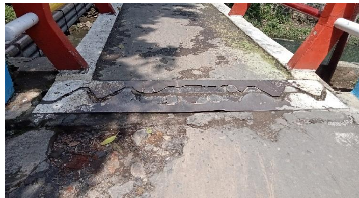
KONDISI EXPANSIONT JOINT
