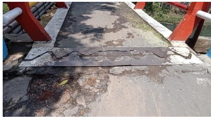
KONDISI EXPANSIONT JOINT
