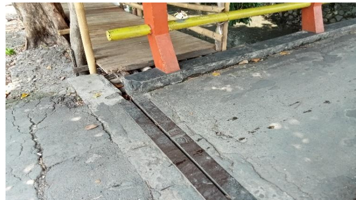
KONDISI EXPANSIONT JOINT
