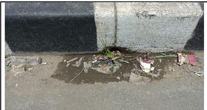
PIPA CUCURAN DRAINASE JEMBATAN
