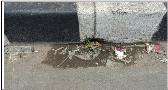
PIPA CUCURAN DRAINASE JEMBATAN
