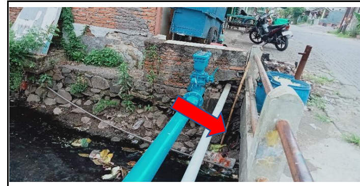
DINDING PENGAMAN TANAH PECAH
