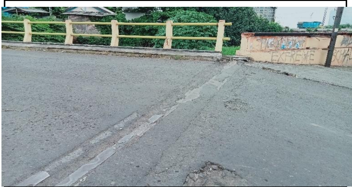
EXPANSION JOINT MENGLUPAS
