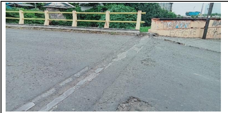
EXPANSION JOINT MENGLUPAS
